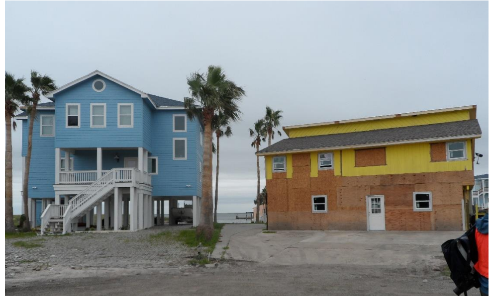
This photo shows examples of different building standards. The left house is elevated and fared well through the storm. The right house is at-grade on a concrete slab, sustained damage during Hurricane Harvey, and thus is boarded up with plywood.
